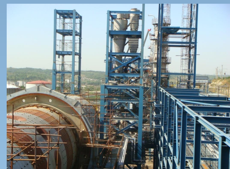
(Above) View of Combustion End and Hydrocarbon Vapour Cyclones.
