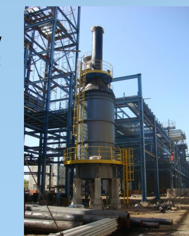
(Right) High efficiency baghouse dust collectors and flue gas fan.
