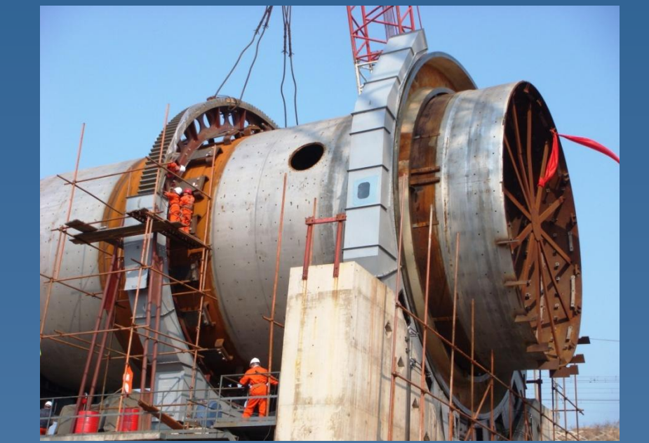
(Above and Left) Assembly of the ATP Processor on the plant site in Fushun, China.
