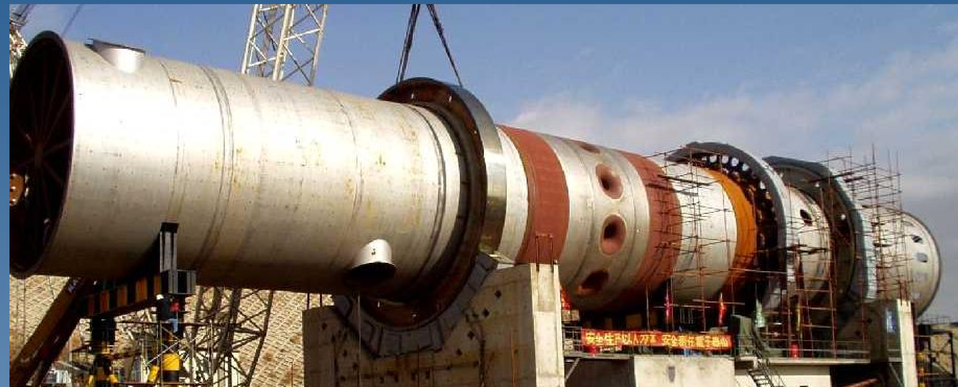
(Above) The ATP Processor for the FMG Project is similar in size to the Processor for the Stuart Oil Shale Research and Development Project, built in Gladstone, Australia in 1999.
