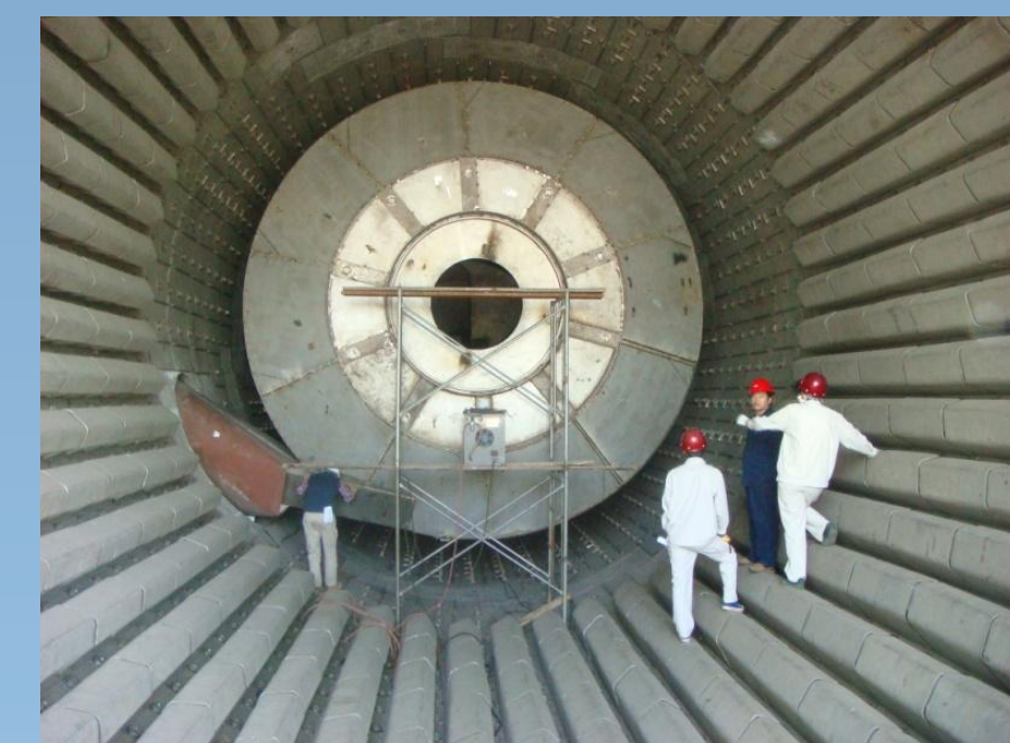
(Above) View inside the ATP Processor Combustion Zone.
