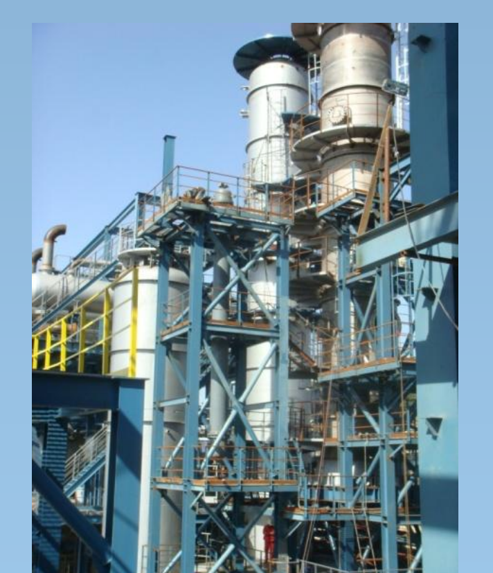
(Above) Oil Recovery plant.
