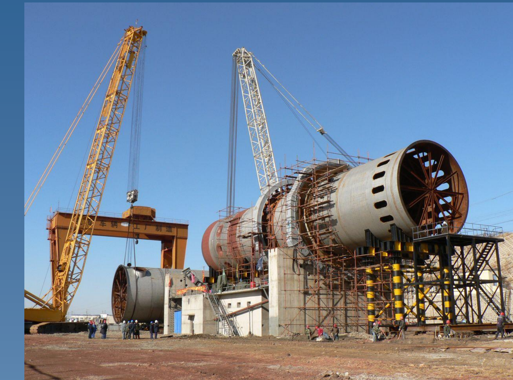
(Above and Left) Assembly of the ATP Processor on the plant site in Fushun, China.
