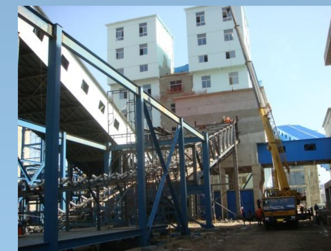
(Above) Feed and Ash Handling Systems.
