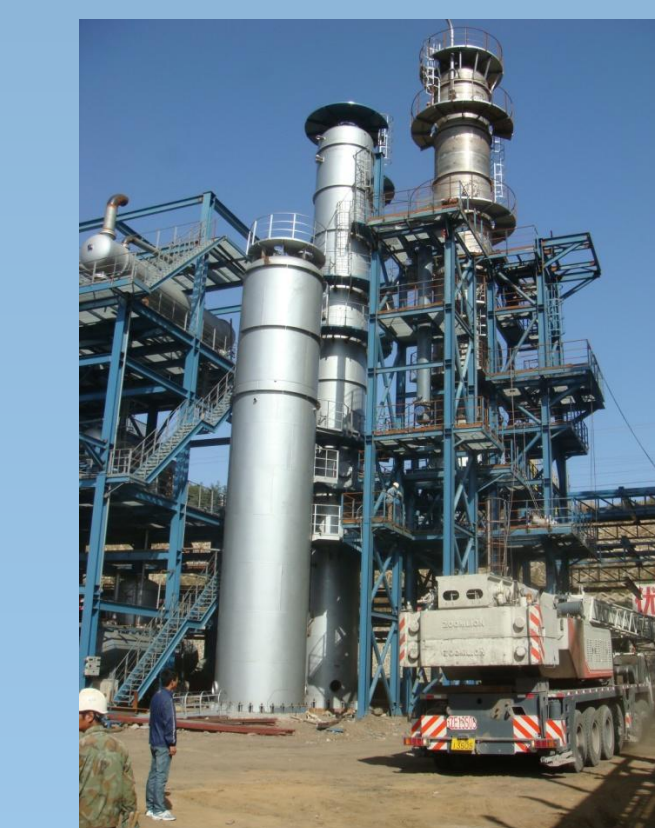
(Above) Hydrocarbon Vapour Scrubber and Fractionator (Oil Recovery).
